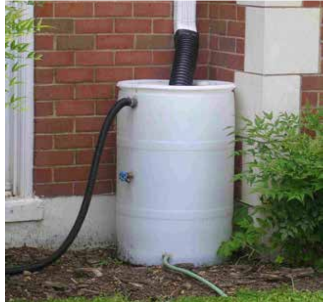
Rain barrels collect roof runoff and the water can be used in your garden.
